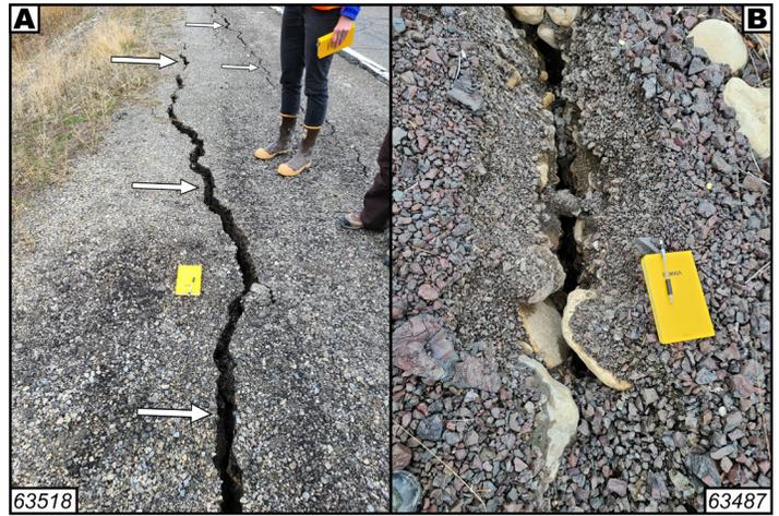
Figure 10. (A) Multiple cracks (shown by arrows) in the roadway base material along the Great Salt Lake State Park Marina Access Road. Primary crack shows approximately 3–4 cm of vertical separation. Field notebook (10 cm wide) for scale. (B) Close-up view showing approximately 30-cm-deep crack. Resource ID from the Magna earthquake online clearinghouse labeled in bottom right corner of photos.
