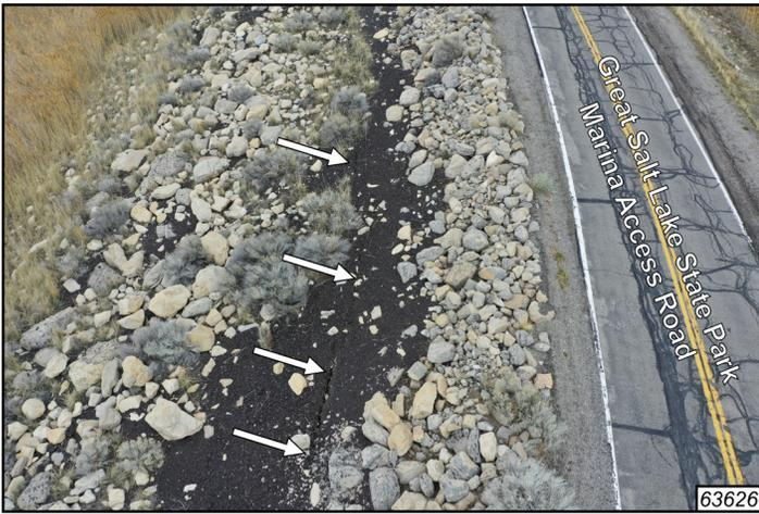
Figure 9. sUAS image of the Great Salt Lake State Park Marina Access Road showing an approximately 6-meter-long crack in the roadway base material (shown by arrows). Resource ID from the Magna earthquake online clearinghouse labeled in bottom right corner of photo.
