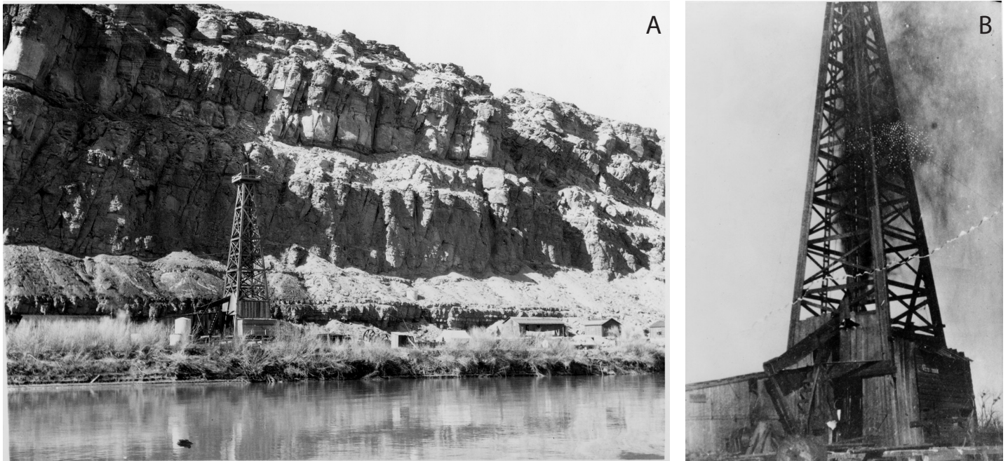
Figure 1. Midwest Exploration and Utah Southern No. 1 Shafer well, drilled in 1924. (A) View across the Colorado River. The cable-tool rig was floated down the river from the town of Moab. (B) The well blew out after encountering gas at 2028 feet (618 m) in the Cane Creek shale and the rig caught on fire and was destroyed. Courtesy of the Utah Division of State History and the Utah State Historical Society.
