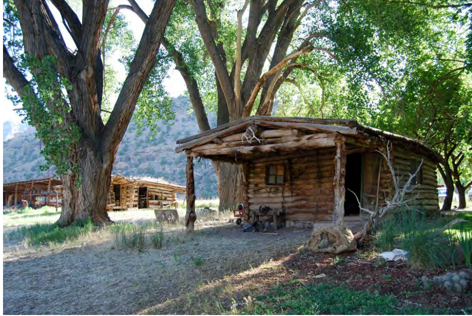
Old work shed at Wilcox Ranch. Photograph by Nora Nieminski.
