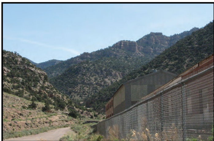
Figure 7. View of Geneva Coal Mine, at the mouth of Horse Canyon, on the right side of the road looking up the canyon.
