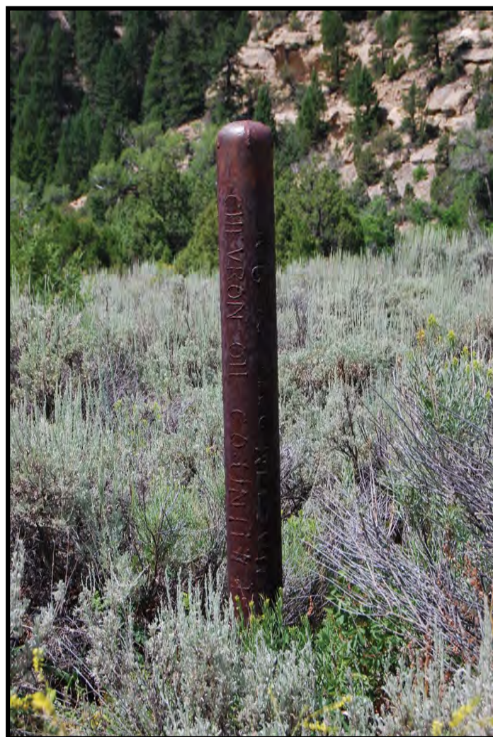
Figure 11. Dry well marker at the mouth of Dry Canyon, capping an abandoned exploratory gas well drilled by Chevron Oil Company in 1974.
