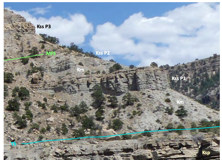
Figure 18. Retrogradational to aggradational parasequences within the Storrs Member (Kss) on the west side of the mouth to Sowbelly Gulch. Ksp and Km refer to the Panther Tongue Member and Mancos Shale, respectively. Parasequences are marked by P1, P2, and P3. The transgressive (TS) and maximum-flooding (MFS) surfaces are shown by a blue and a green line, respectively.
