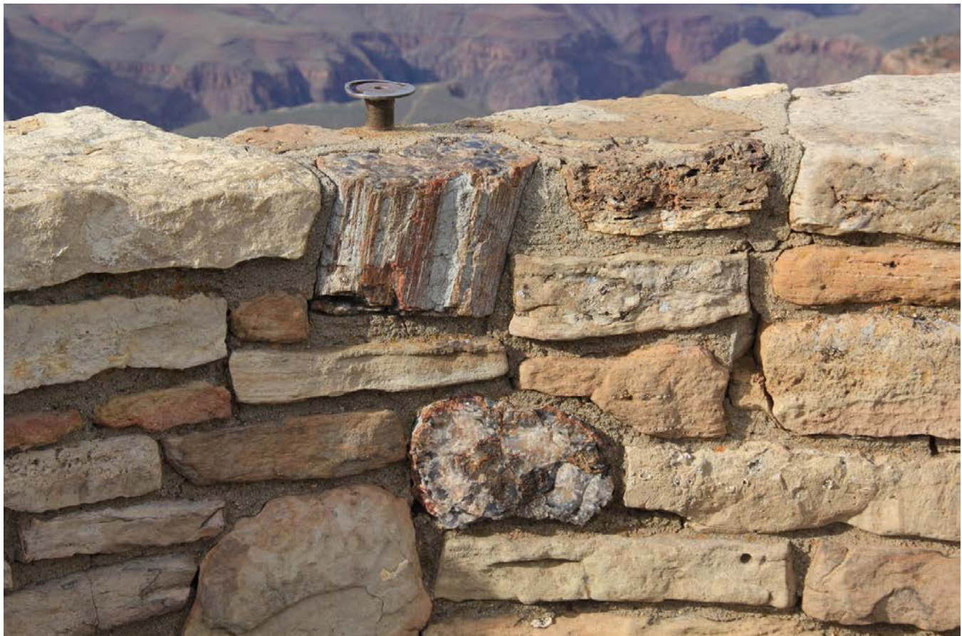
Figure 17. Two large chunks of petrified wood used as building materials for the wall along the Rim Trail outside the Verkamp's Visitor Center on the South Rim (NPS/DIANA BOUDREAU).
