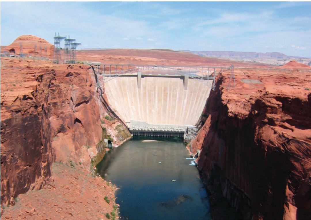
Figure 6. Glen Canyon Dam, Arizona, which forms Lake Powell, is built into the Navajo Sandstone, Glen Canyon National Recreation Area, Utah and Arizona.
